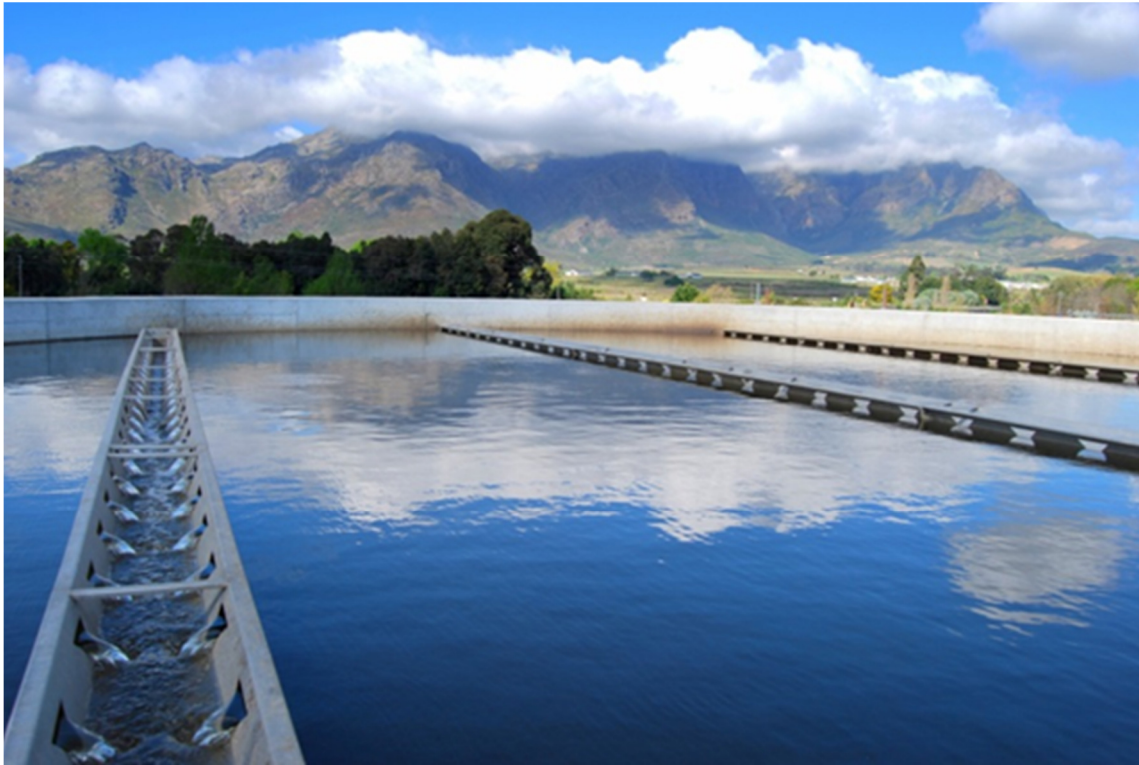
Figure 10. Nereda ® reactor at Wemmershoek discharging effluent.
