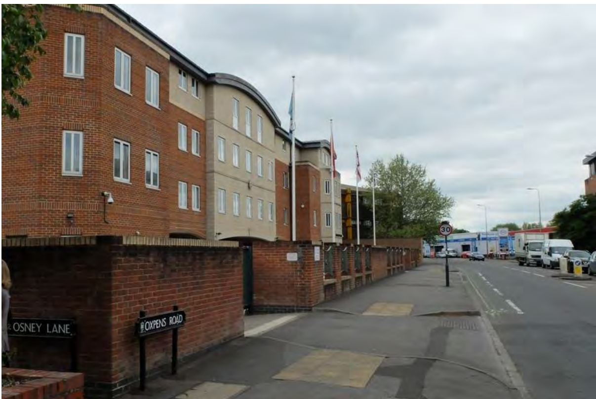
Not far from the city centre, The Oxford University Royal Naval Unit seems to show how far the public sector commissioning process has moved away from a culture which produced the exquisite architecture of the Royal Naval College at Dartmouth
