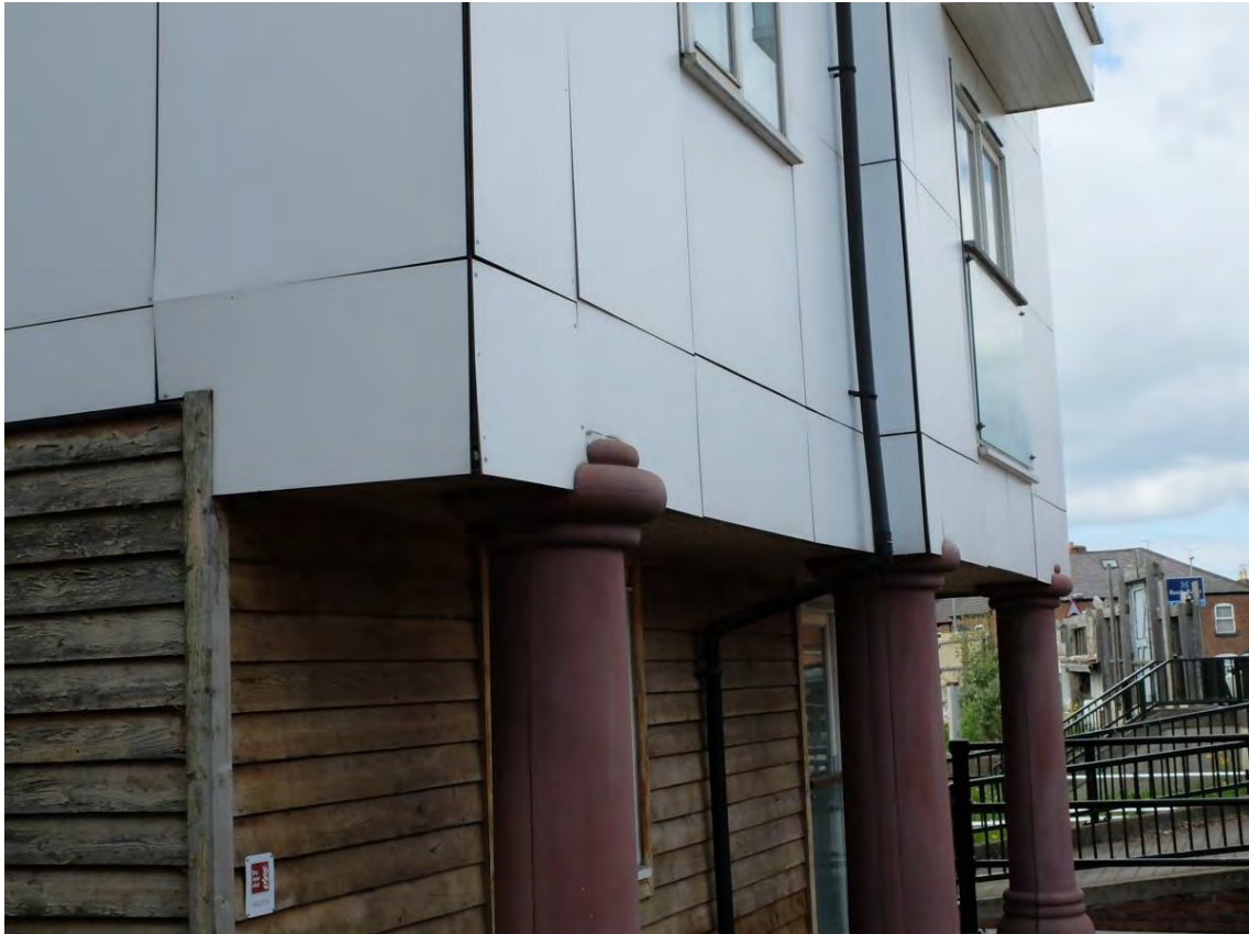
Some materials and detailing are questionable
