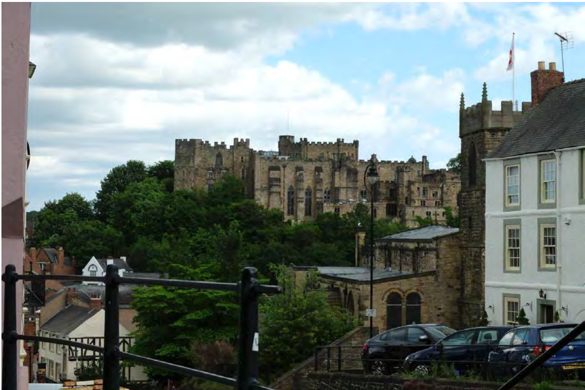
The west walls of Durham Castle from Crossgate
