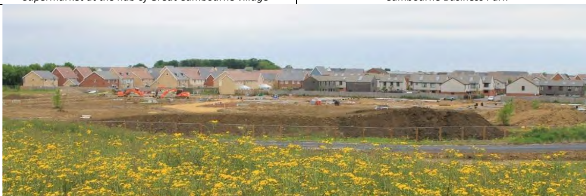
Development in progress at Upper Cambourne seen from Broadway, the eastern edge of the new village
