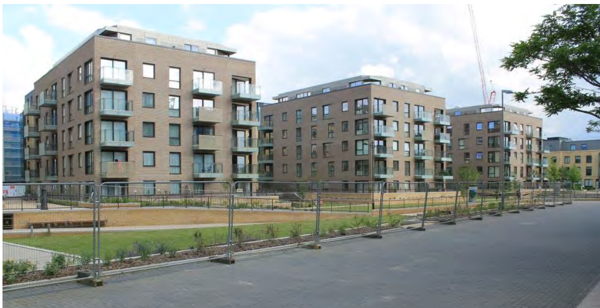
Apartment blocks in the CB1 development near the railway station, with the gardens too almost complete.
