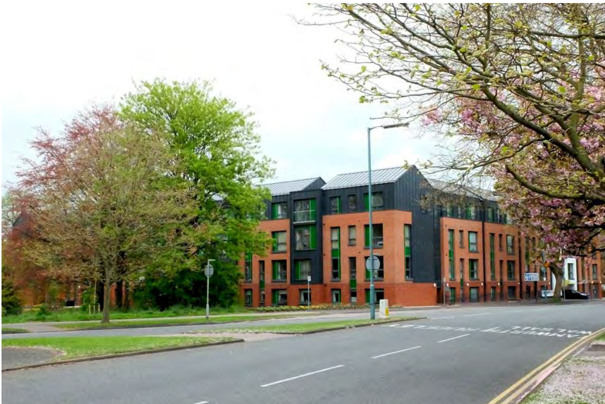
Figure 12 Development on local authority-owned land, Lichfield
